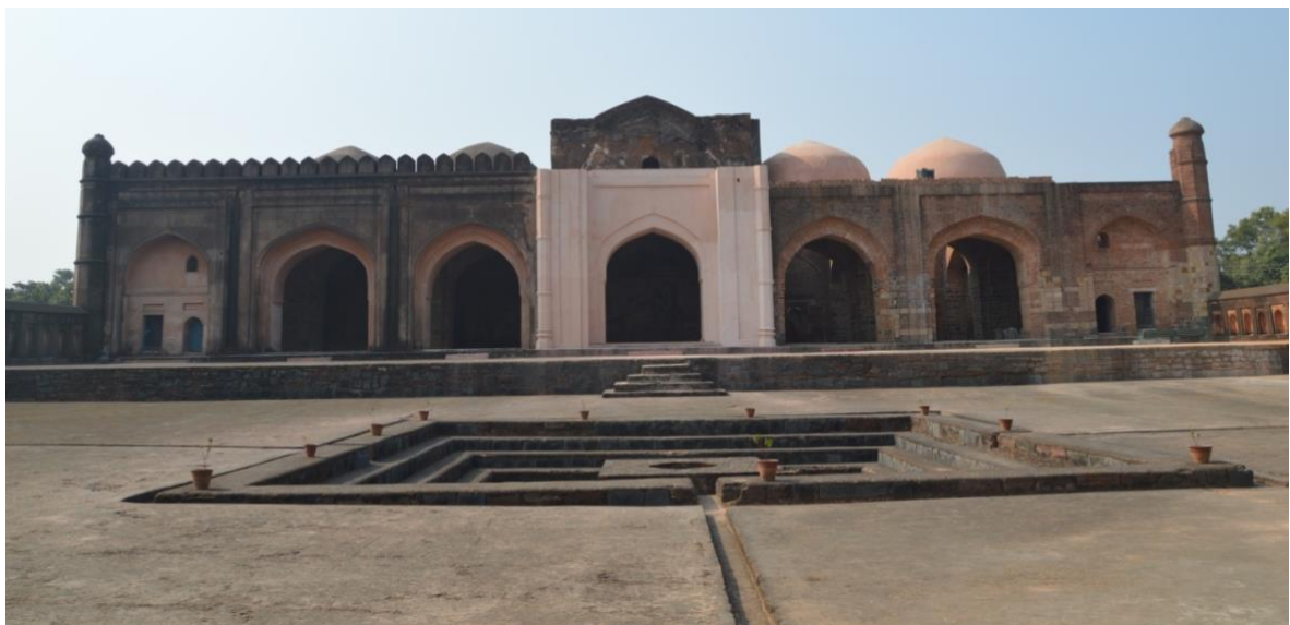
Jami Masjid with some restoration work underway as on 27.12.2020
